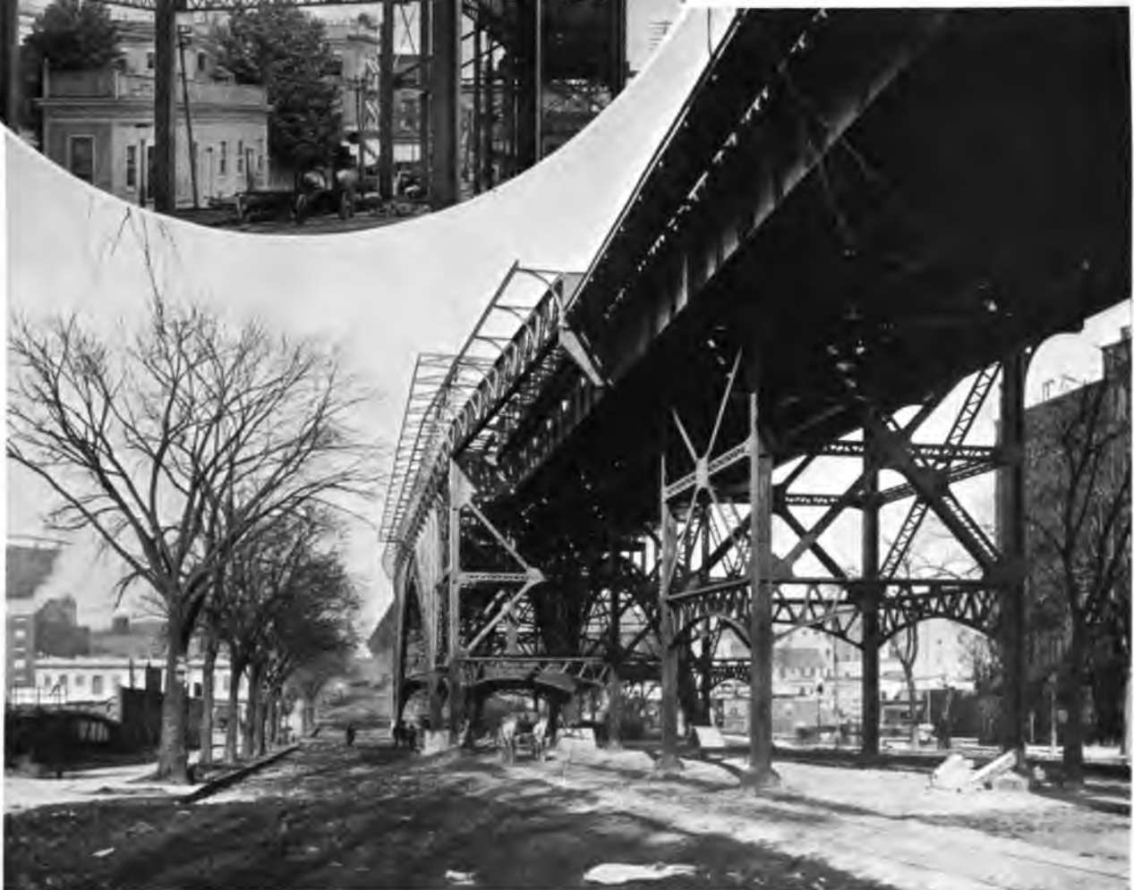
MANHATTAN VALLEY VIADUCT, LOOKING NORTH
